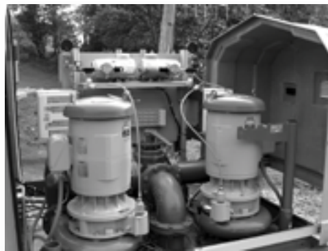
New pumping equipment was installed at the Lunt Road pumping station.
